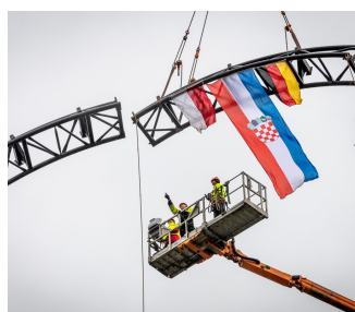
Final rail milestone: The final rail element is 6.71 metres long and weighs 1.9 tonnes
