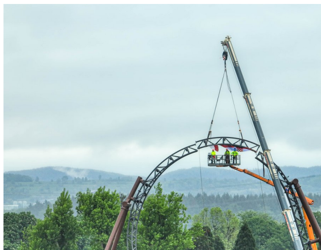
Final rail milestone: The final rail element is 6.71 metres long and weighs 1.9 tonnes
